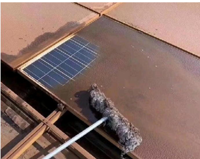
Fig. 2: Dust fall on solar panels.
