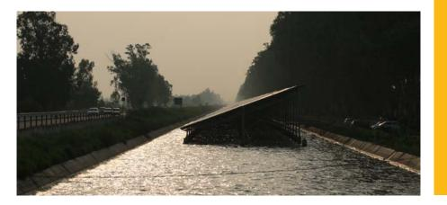
in Asia. The EPC contractor for the projects was PES Engineers Private Limited, who installed 16,680 REC Peak Energy 72 solar panels on on two spreads, including over 1.25 km from Rajgarh to Ajnod village downstream on Sidwhan canal..
