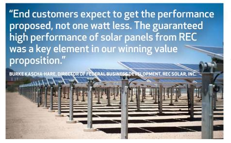
The 4.5 MW installation comprises a 2.9 MW carport roof system and a ground-mounted 1-axis tracker installation of 1.4 MW. While the carport system serves the dual purpose of generating power and providing shade, the tracker was installed on dormant land that was not ideal for any other use. In all, the installation consists of 19,526 solar panels, of which 18,154 are REC 235W PE-US (carports) and 1,372 are REC 220W PE.
