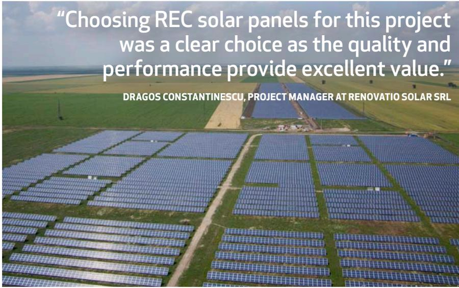
**ROMANIA'S CURRENT LARGEST SOLAR POWER PLANT** is powered by 41,760 solar panels from REC. Located in Giurgiu County in southern Romania, the 10 MW Izvoru Photovoltaic Park is owned by Power Live One Srl and was built by Romanian EPC company Renovatio Solar SRL.
